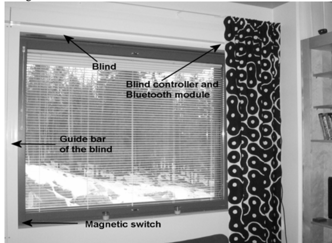
Figure 7: The components of the controllable blinder.
